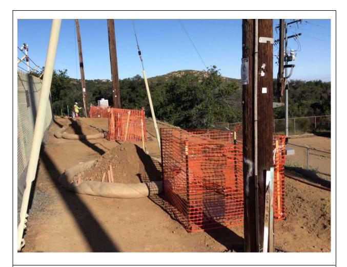
**Photo 4:** Spoils from pole excavations occurring along TL 629A were stabilized with fiber rolls in accordance with the Erosion Control Plan and SWPPP (MM HYD-1, MM BIO-7) and excavations were securely covered in accordance with MM BIO-23.
