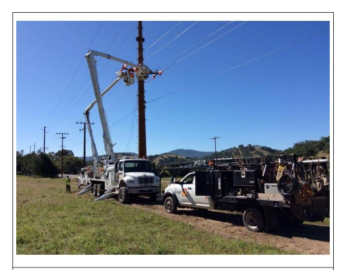
**Photo 5:** A construction crew was observed removing temporary disconnects at Pole Z128035 on TL 682. Construction work occurred within the work limits and approved access road in accordance with MM BIO-1.
