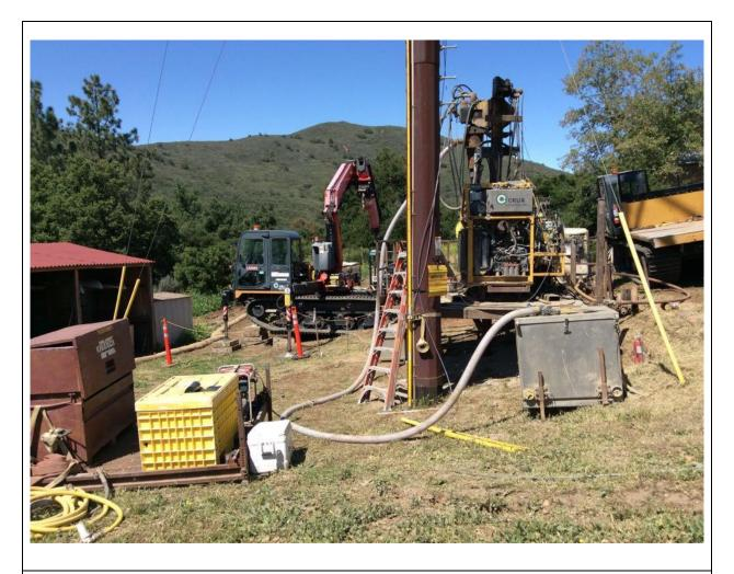
**Photo 2:** A containment box was used to trap drill cuttings during micropile drilling in order to reduce dust emissions at Z173104 (TL 629A) in accordance with APM AIR-05. Fuel for the micropile equipment was observed stored within a double-walled cell to prevent the release of hazardous materials onto the ground in accordance with MM PHS-2.
